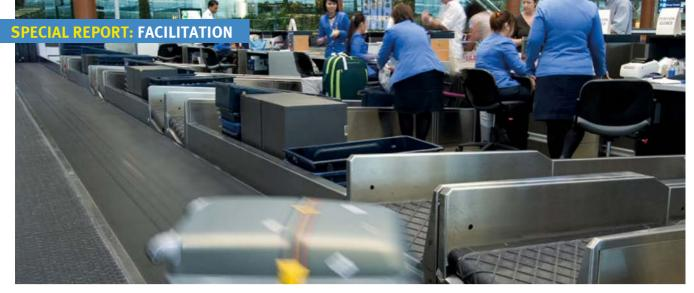
For ICS however, unscreened baggage is loaded directly into individual containers (tubs) at the ticket counter load points, collected onto delivery mainline conveyors and transported to a pre-CBIS bag storage/screening load levelling facility. The number of scanners and screening stations is the same, in part due to the pre-CBIS bag storage.
